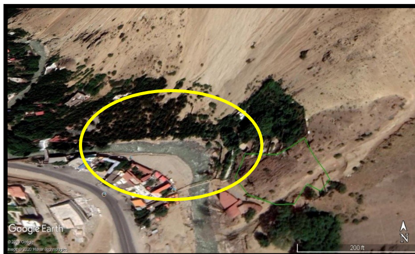
Figure 12. Construction on the riverbed (Dimension 1116X632, Width 1116 pixels, height 632 pixel, Resolution 96 dpi; Imagery Date: 06/30/2019; 35° 50' 38.93" N 51° 33' 34.83" E elev 5684 ft eye alt 6218 ft).
