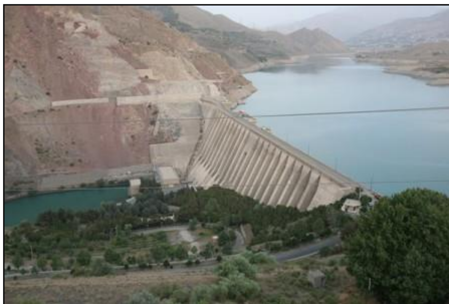
Figure 4. Latyan Dam Lake
