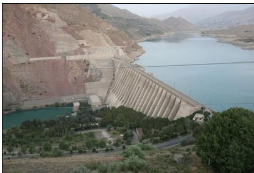
Figure 4. Latyan Dam Lake
